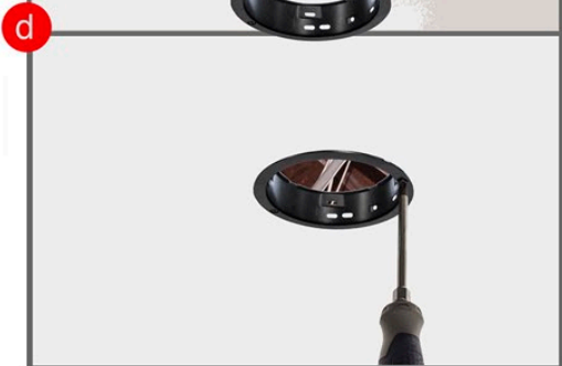
Step C- Install ceiling and cut opening. Paint drywall. Slide flange receiver into opening. Step D- Tighten screws to clamp receiver to ceiling.
