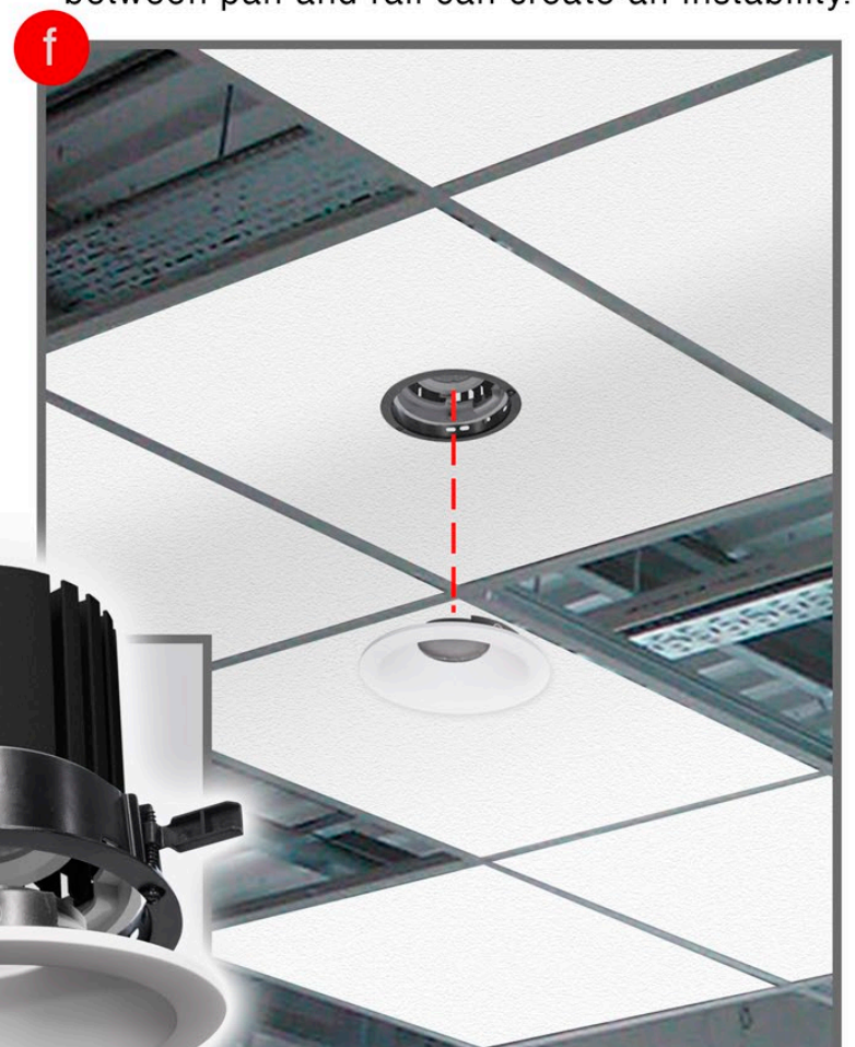
Step C- Check to see that dropped pan is resting securely on top of tile rails. Any gap between pan and rail can create an instability.
