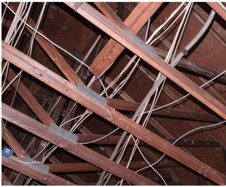
Exposed Ceiling Joists
