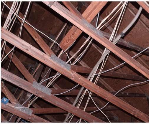
Step 1- Exposed Ceiling Joists
