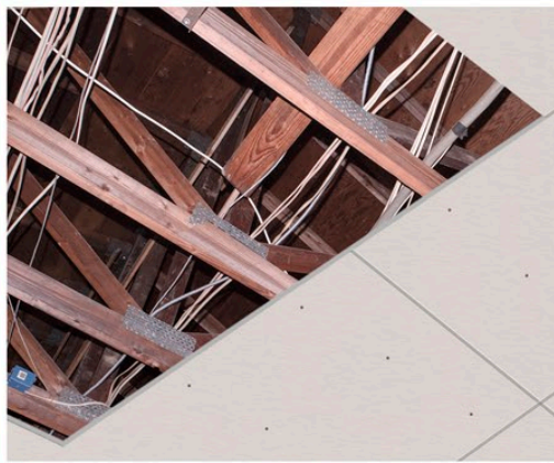
Step 2- Install GWB ceiling.
