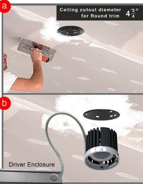
Step 4a- Plaster over receiver Step 4b- Connect main electrical wiring to lighting fixture
