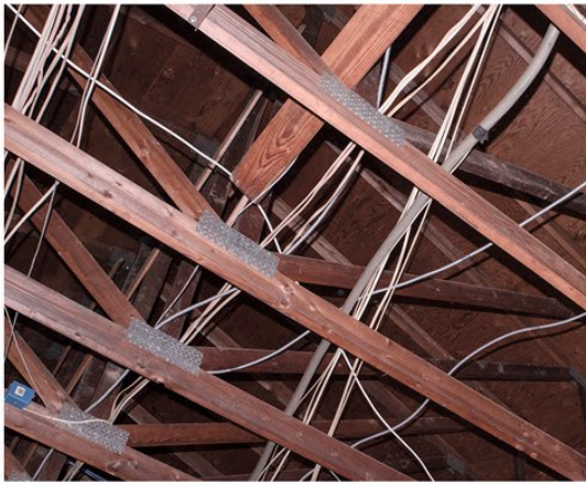
Step 1- Exposed Ceiling Joists
