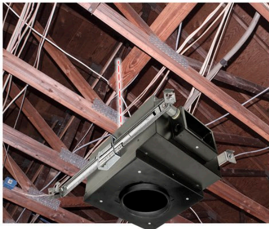
Step 2- Adjustable Mounting Rails anchor housing to ceiling joists with screws
