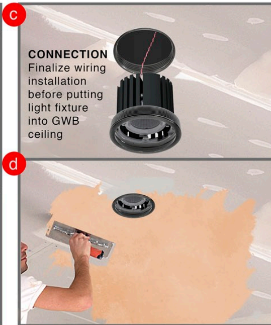
Step 4c- Finalize wiring, screw receiver with attach light fixture into housing. Step 4d- Apply tape and joint compound (dry). Plaster over GWB ceiling
