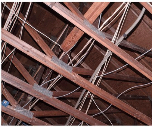
Exposed Ceiling Joists
