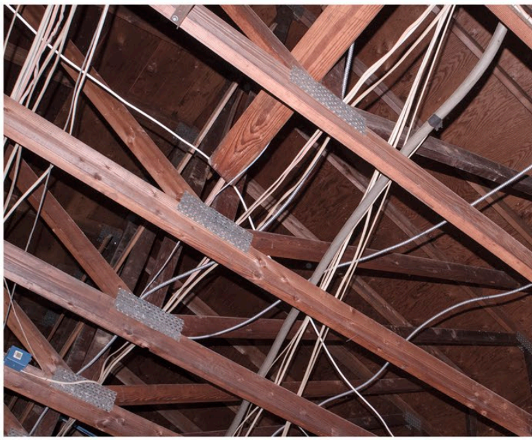
Step 1- Exposed Ceiling Joists
