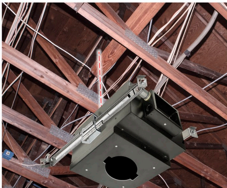
Step 2- Adjustable Mounting Rails anchor housing to ceiling joists with screws
