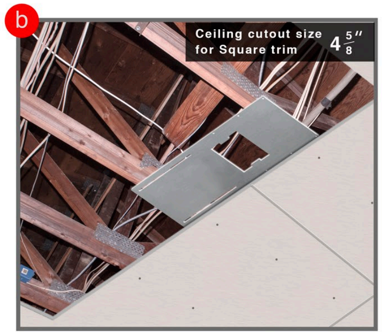
Step B- Place GWB over new pan.
