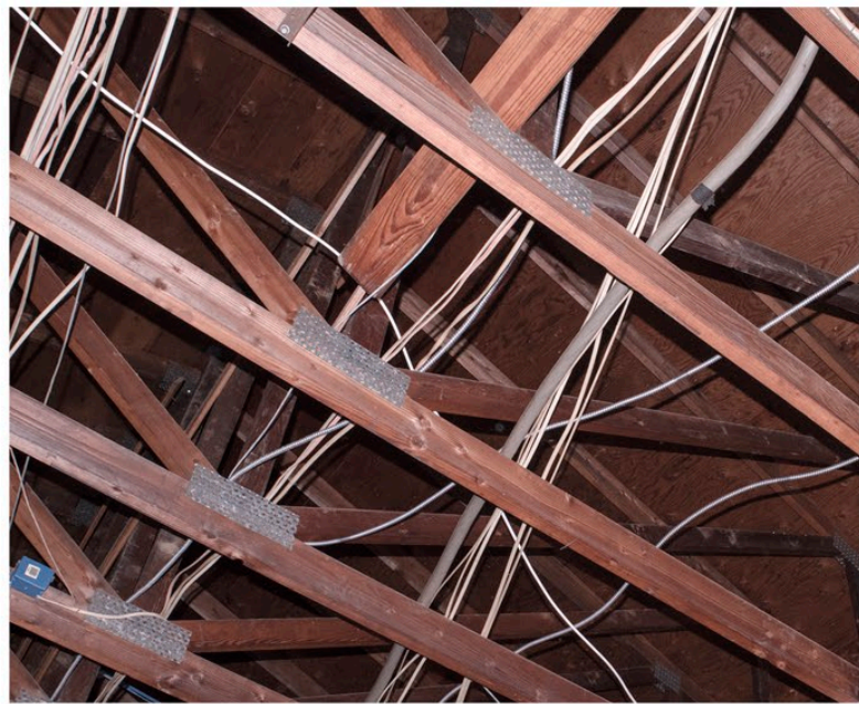
Exposed Ceiling Joists
