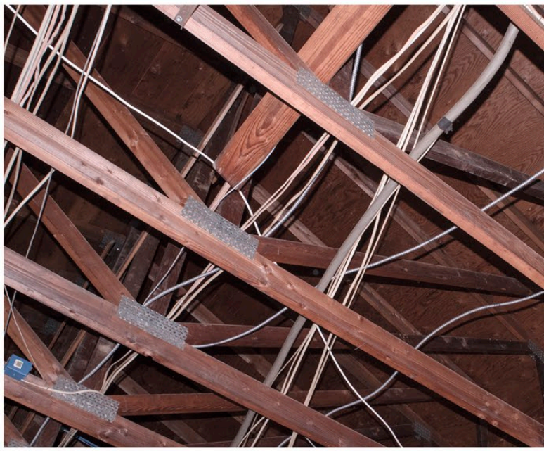
Exposed Ceiling Joists
