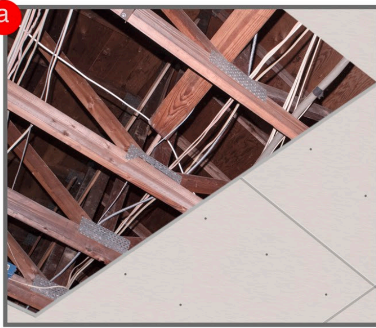
Step A- Install ceiling.
