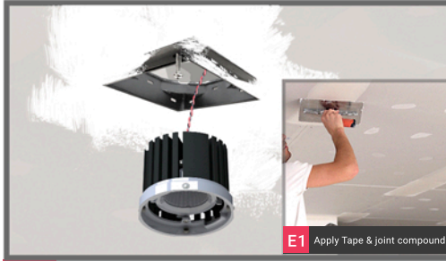
E Plaster receiver flange. Finish electrical
