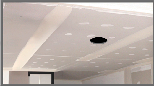
C Cutout opening for light install.
