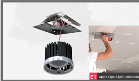
E Plaster receiver flange. Finish electrical
