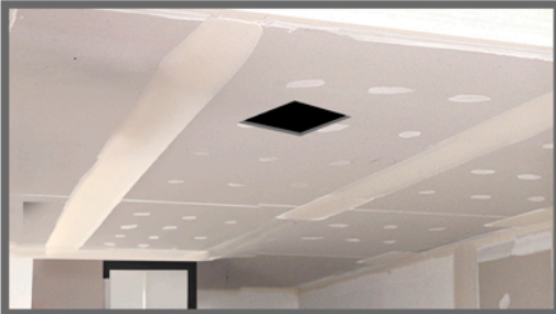
C Cutout opening for light install.
