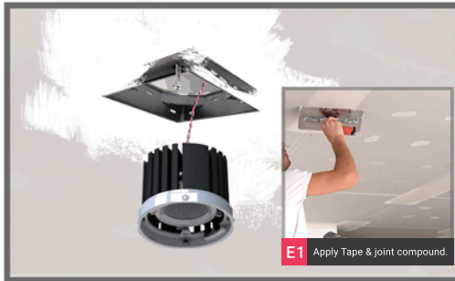
E Plaster receiver flange. Finish electrical
