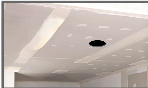
C Cutout opening for light install.
