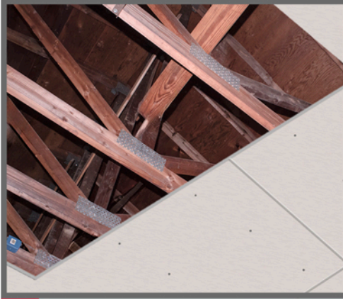
A Install ceiling.
