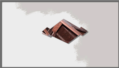
C Paint over ceiling before installation.
