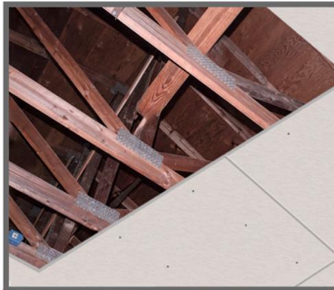
A Install ceiling.
